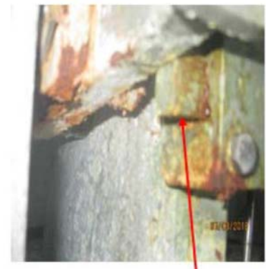
Incorrect setting of safety interlocks
